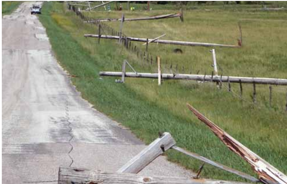
High winds on June 27 brought down 32 poles causing an estimated $500,000 in damages.
