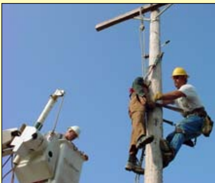
Brian Smylie performs a pole top rescue and John McMillan is in the bucket, ready to assist.
