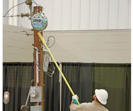
A lineman prepares to demonstrate the effects of Mylar balloons on power lines.
