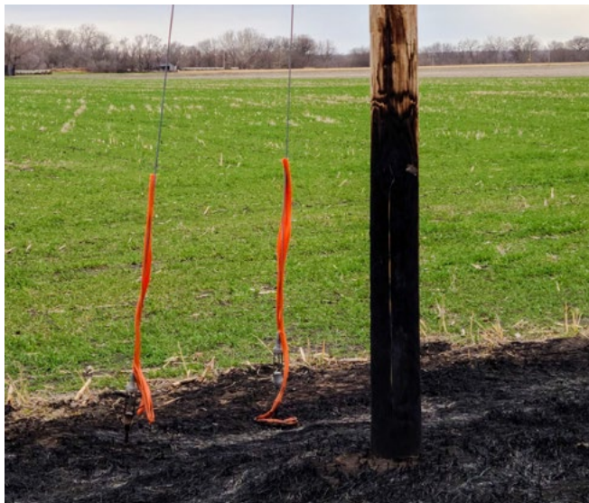
Caney Valley reminds members to plan your burning before you begin. It is much cheaper to prevent a pole from catching fire than to pay for a new pole.
